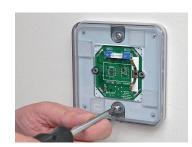
4. Adjust range and delay before activation by turning potentiometer using Philips screwdriver.
